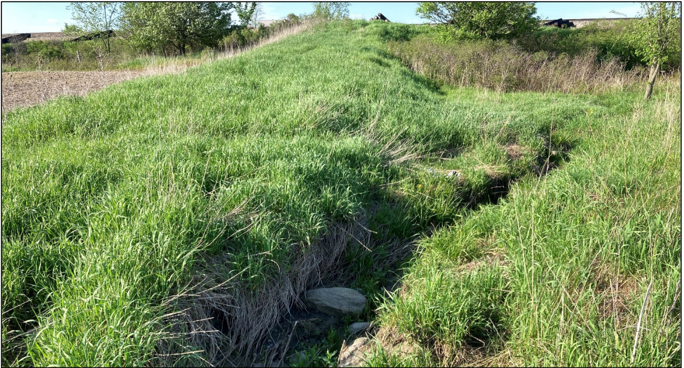
Photo 5: Facing upstream on the dry watercourse channel at the base of the artificial earthen ramp to the railway, near where it exits the site. Note the miniscule channel dimensions.
