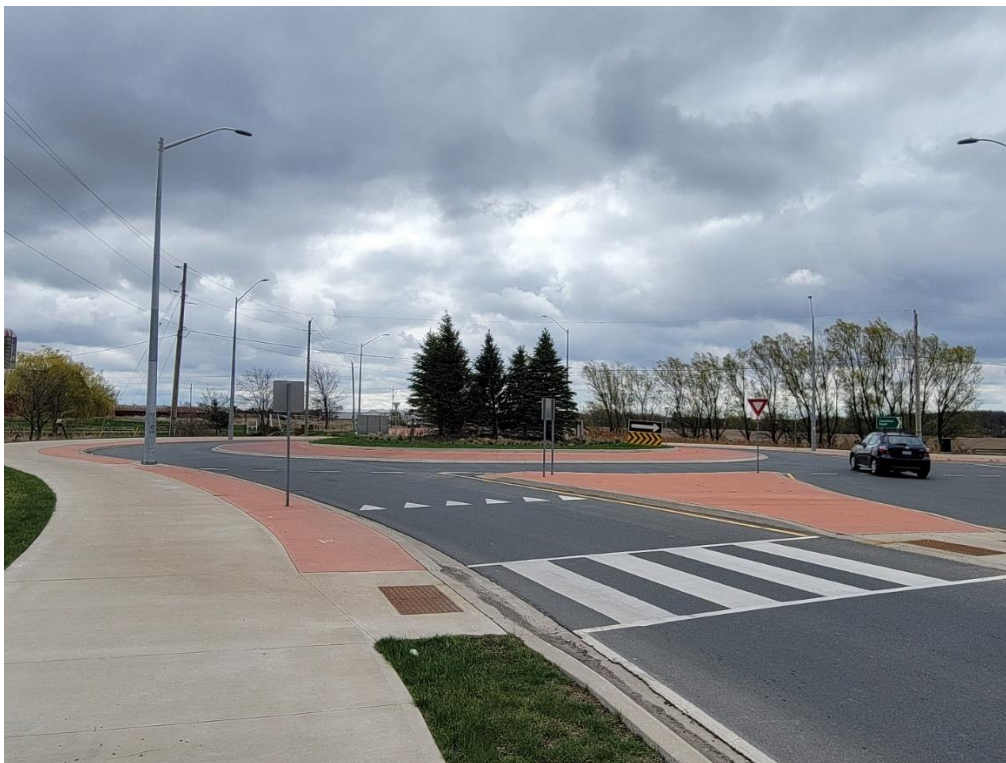
Photo 11 – Roundabout where Townline Road and St. Catharines Street intersect (Location of anticipated street access to Subject Lands)
